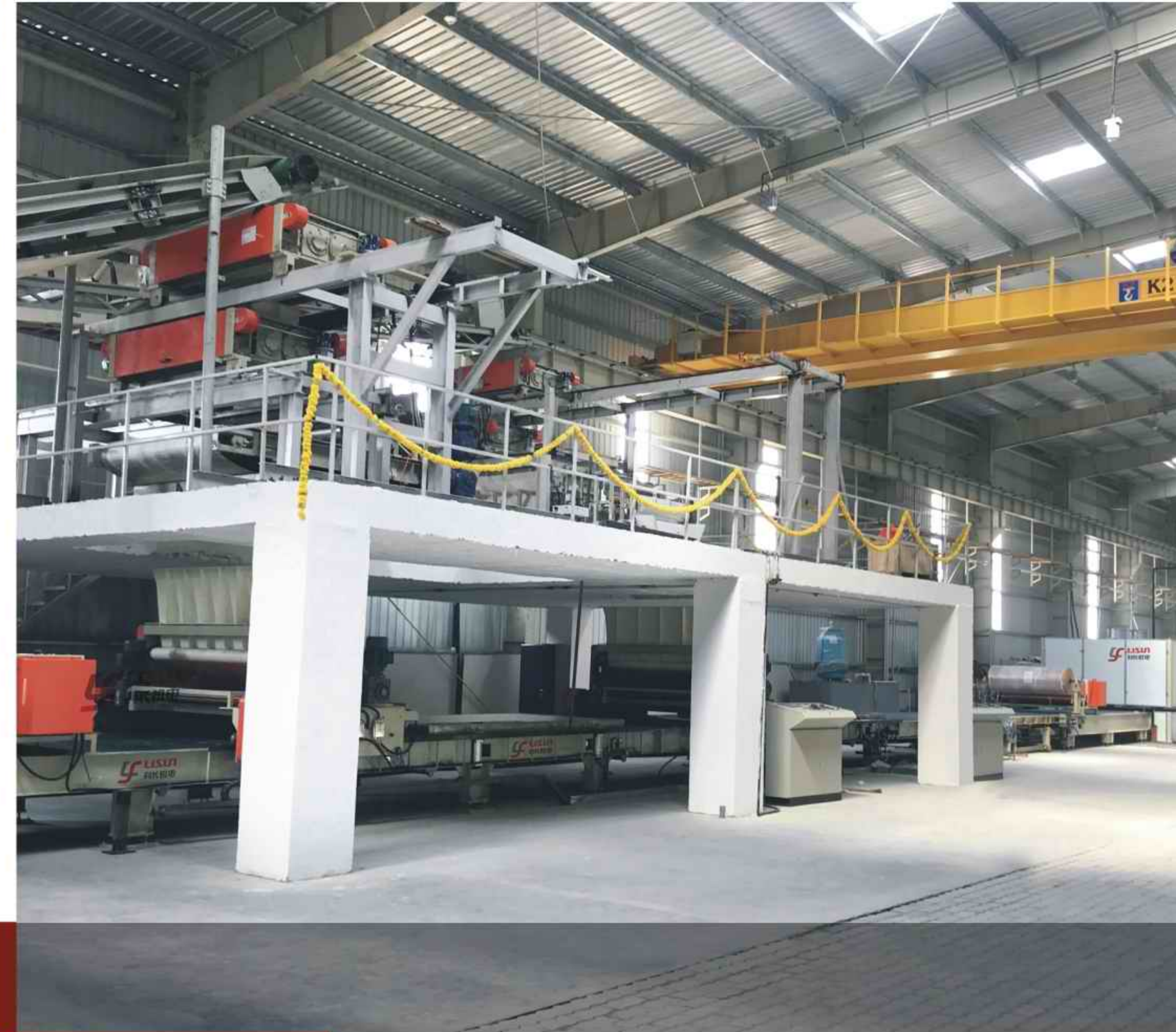
▼ 搅拌、布料系统 Material Mixing / Distribution System
